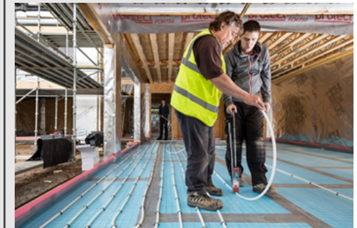
WMS AmbiTak System installation.
