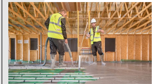
The most common method of incorporating WMS UFH into a new build home is to include the pipework within the floor screed.
